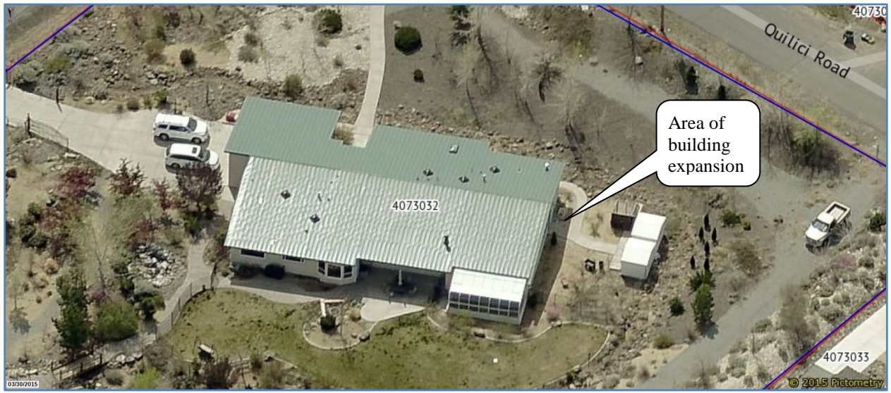
Photos – Existing Conditions
